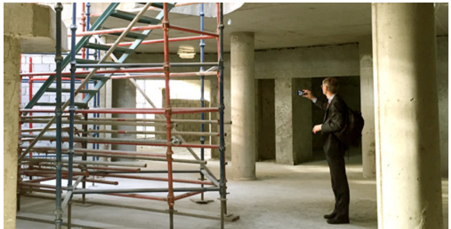
Prof Stammberger during a tour of the TSESI building project in Dubai, April 2018.
