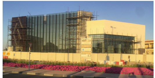
Final construction touch-ups of the TSESI project.
