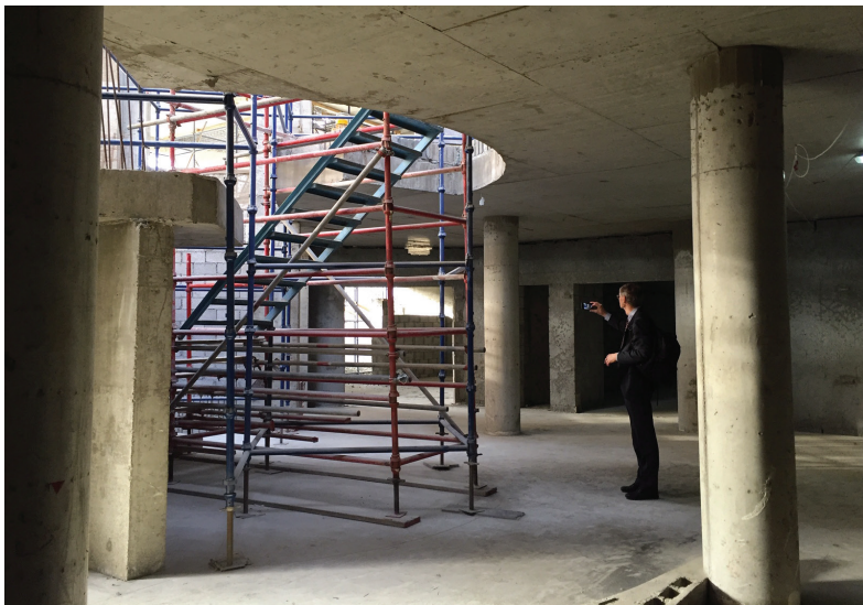
Heinz following up on construction of the TSESI and inspecting progress in spring of 2018.
