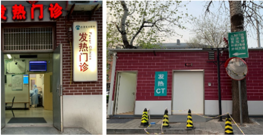
Figure 2. The fever clinic of Beijing Friendship Hospital is in a separate building with the independent consulting rooms, a laboratory for the flu screening test and CBC, an observation room, the isolation rooms and the separate CT room.
